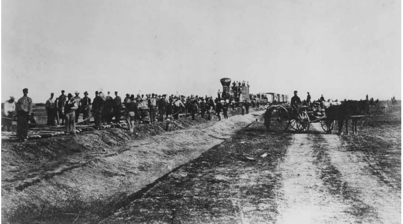
Alexander Gardner took this photograph of workers laying track on the Union Pacific Railroad, Eastern Division, west of Hays, Kansas, dated 1867. When the Kansas Central Railway commenced construction in 1871, the track construction crew consisted of men of mostly Swedish and Irish heritage.
